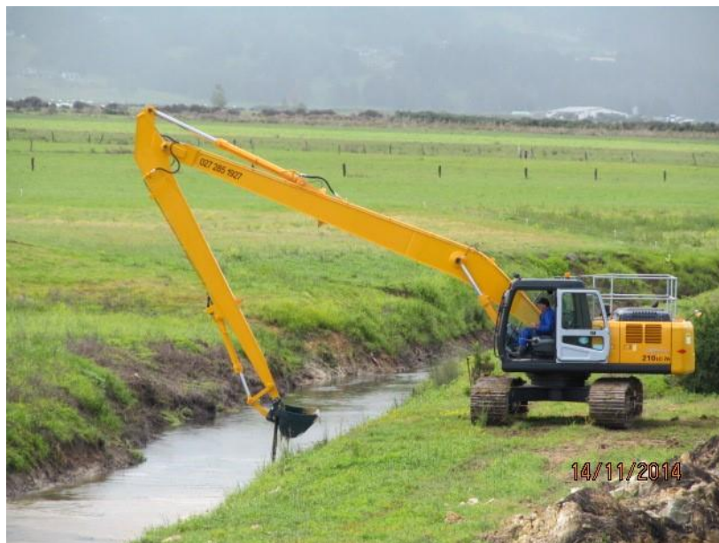
Figure 16: Drain clearance activities in the Hikurangi Repo. (Photo: Whangārei District Council).
