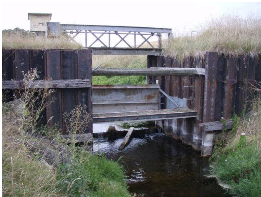
Figure 2: The weir on Poukawa Stream. The radial gate has been lifted, and lake level is being maintained by the horizontal boards. A small flow can be seen overtopping these boards.
