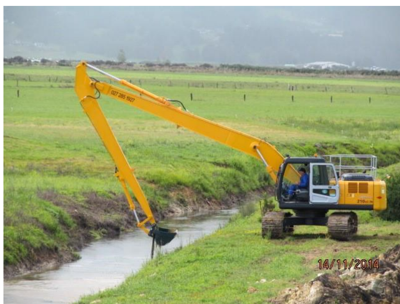
Figure 19: Drain clearance activities in the Hikurangi Repo. (Photo: Whangārei District Council).
