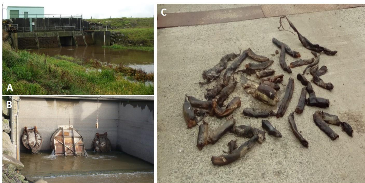
Figure 18: Examples from the Hikurangi Swamp Scheme. (A) A pump station inlet; (B) Flood gates on a pump station outlet; and (C) Some of the tuna killed by one of the Hikurangi pump stations during a flood event in March 2017. (Photos: Jacques Boubée, Alan Halliday). For more information about this particular tuna mortality event, see https://www.maoritelevision.com/news/regional/whangarei-water-turbines-kill-eel-numbers .
