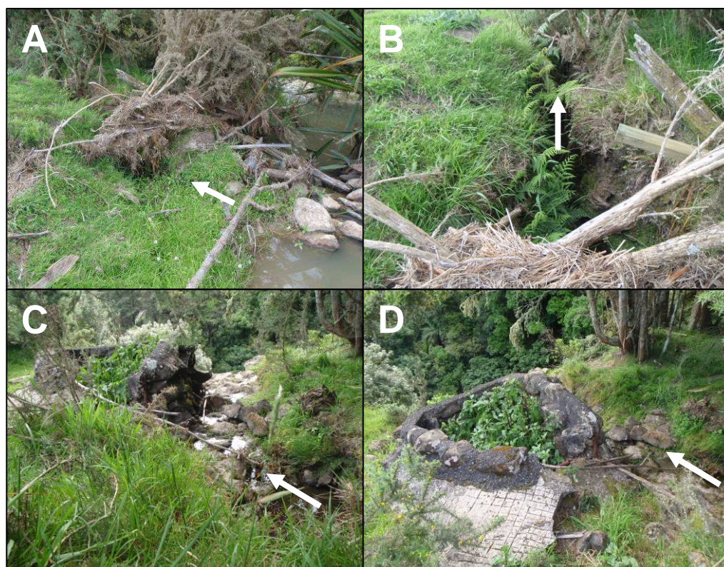
Photo 2. Rock and cement migrant tuna trap on the Utakura River. (A) Small side channel that diverts water from the Utakura River during floods towards the trap; (B) Side channel; (C) Upstream view of approach to migrant tuna trap; (D) Migrant tuna trap. Arrows indicate flow pathway and direction. (Photos: Erica Williams).
